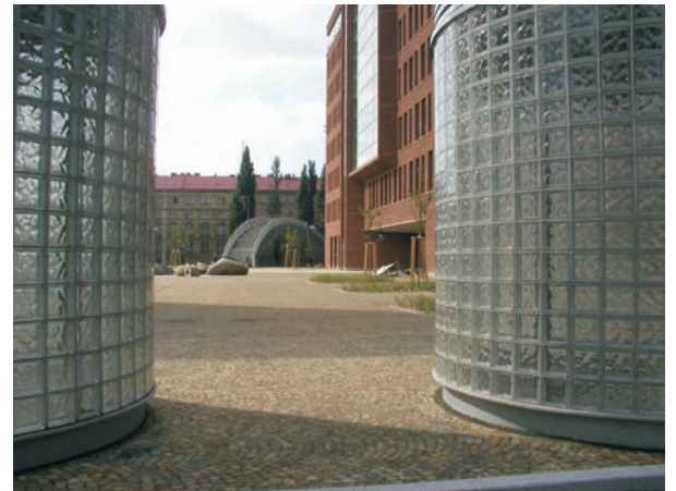
Pedestrian connection downtown with the riverbank build on a light bridge, based on diaphragm wall
