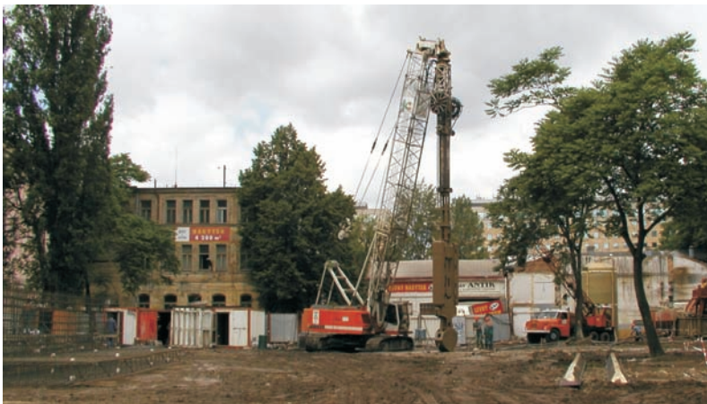
The bridge base works, by excavator with grab 600 mm wide.
